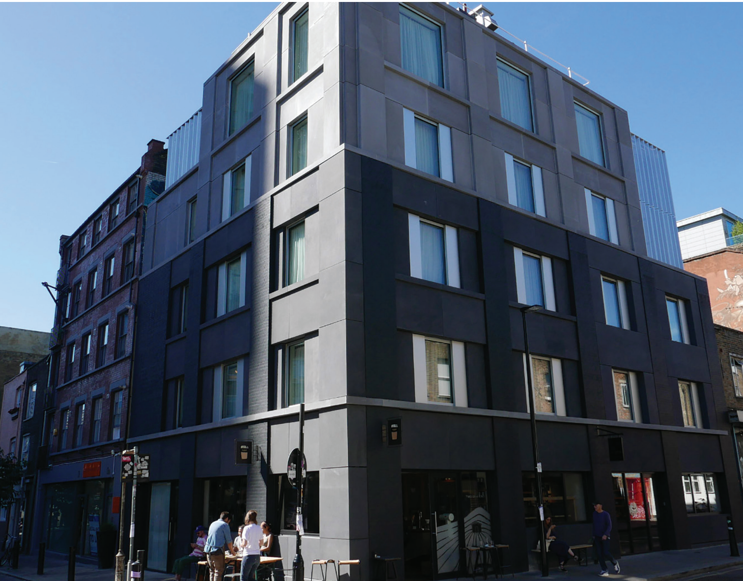
1423 RED CHURCH CORNER, LONDON Black and Charcoal Grey Jesmonite AC730 panels by Alpha Structures
