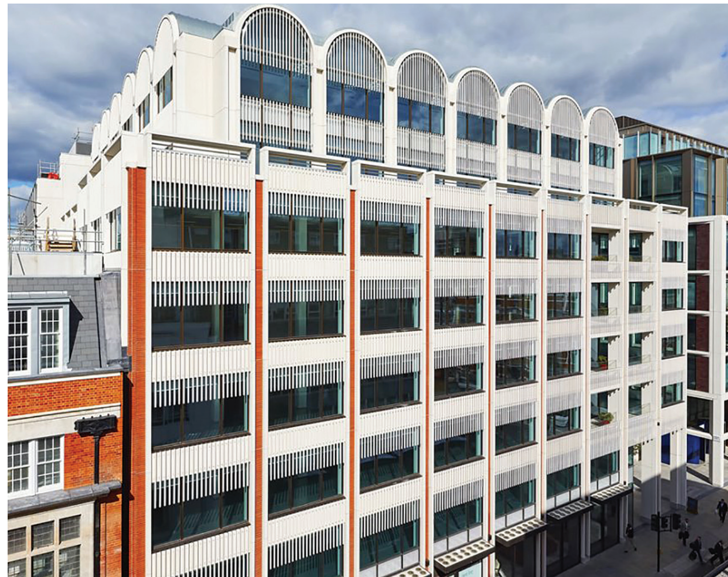
FITZROY PLACE, LONDON Jesmonite AC730 tubular Brise Soleil by Simplicity Abutments
