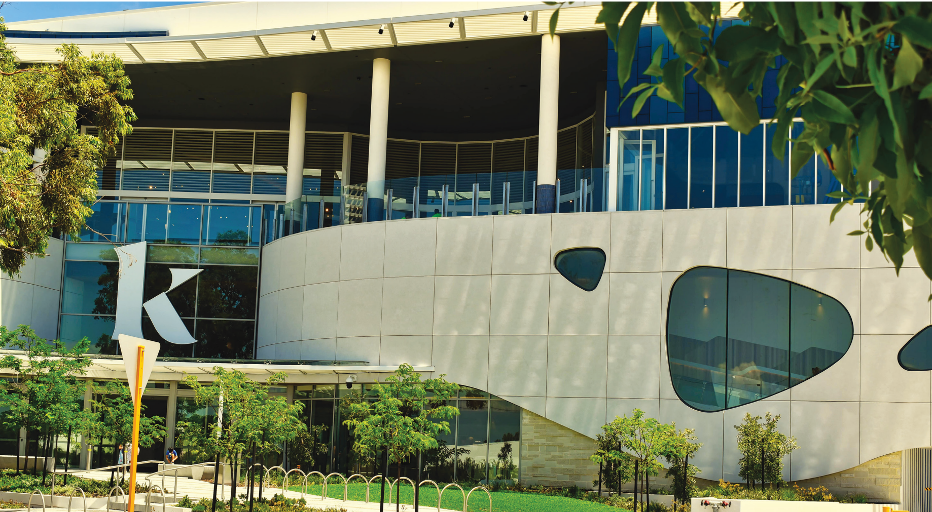
Karrinyup Shopping Centre Expansion Project, AMP Capital Jesmonite AC730 Silver Grey Granite Manufacturer - HGN Design Architect - Hames Sharley Builder - Multiplex
