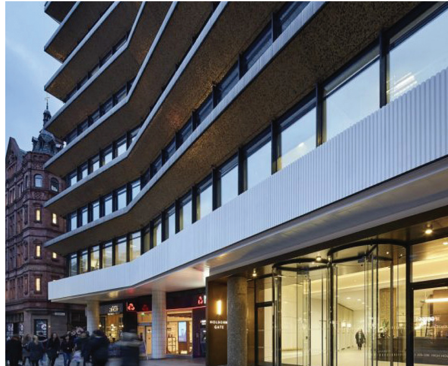
HOLBORN GATE, LONDON Exterior cladding detail Jesmonite AC730
